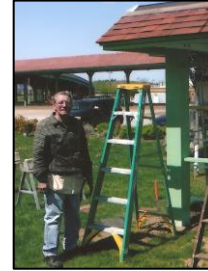
Fred constructing the LH Kiosk in La Porte
